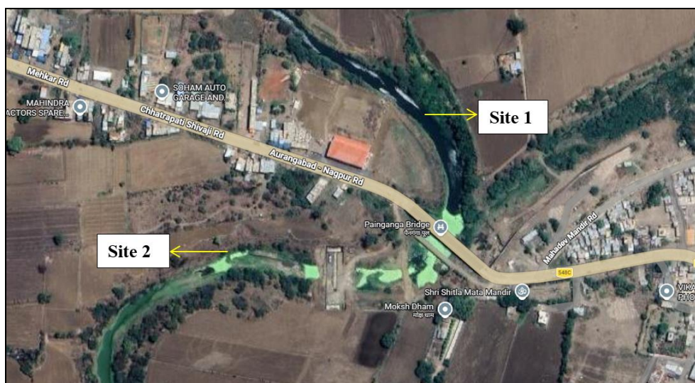
Fig 1: Satellite view of Painganga river bridge of Mehkar Tehsil of Buldhana District
